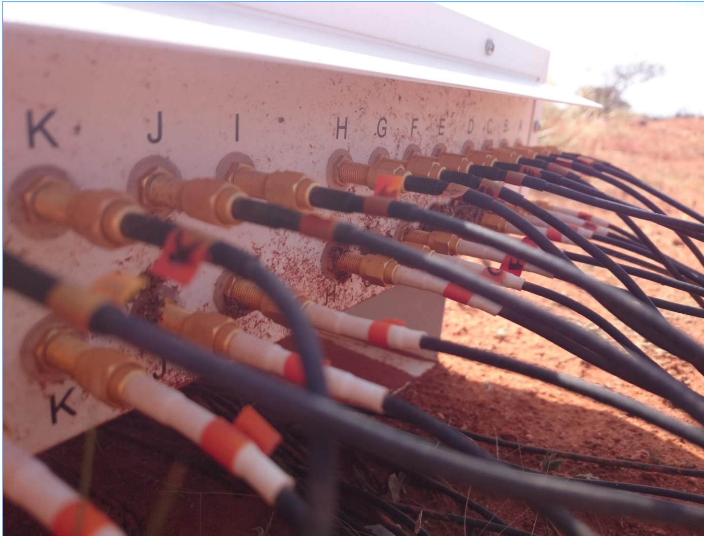
April 2017: There was evidence of a higher water flood level on multiple beamformers in the Southern hex.
