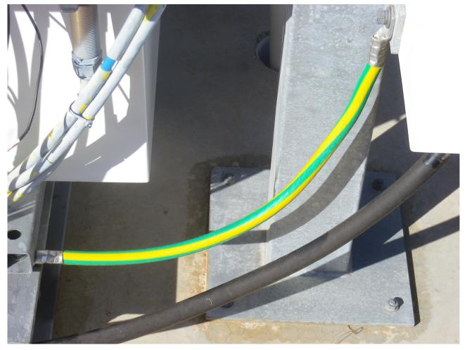
Figure 1: New and improved thick copper earth wire
