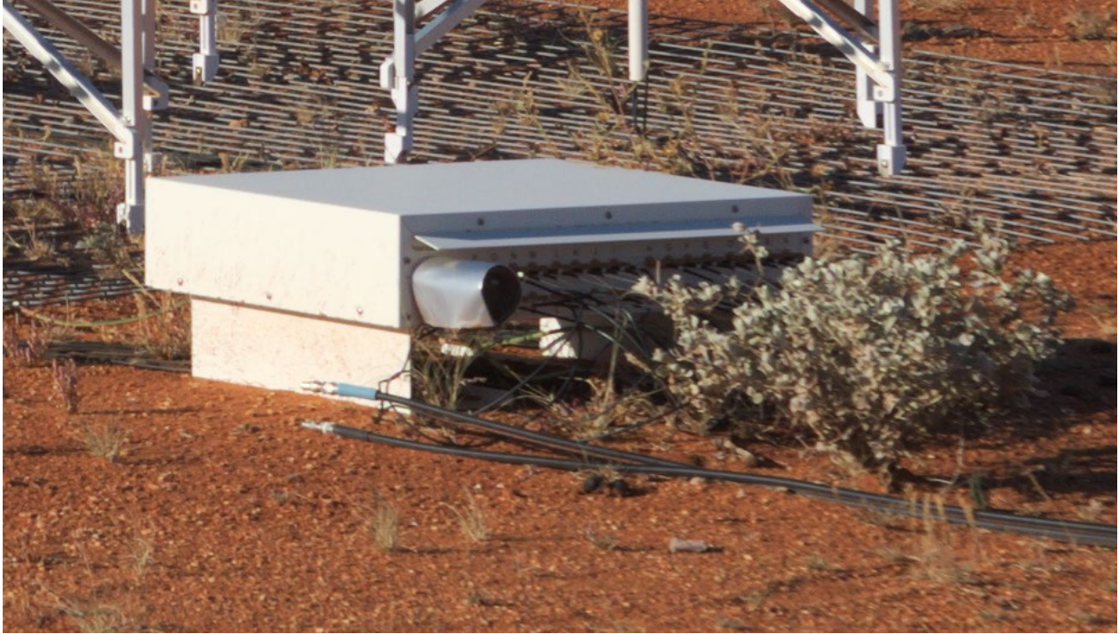
FIGURE 1: SHOWING HAND-FOLDED COVER OVER LIGHTNING ARRESTORS
