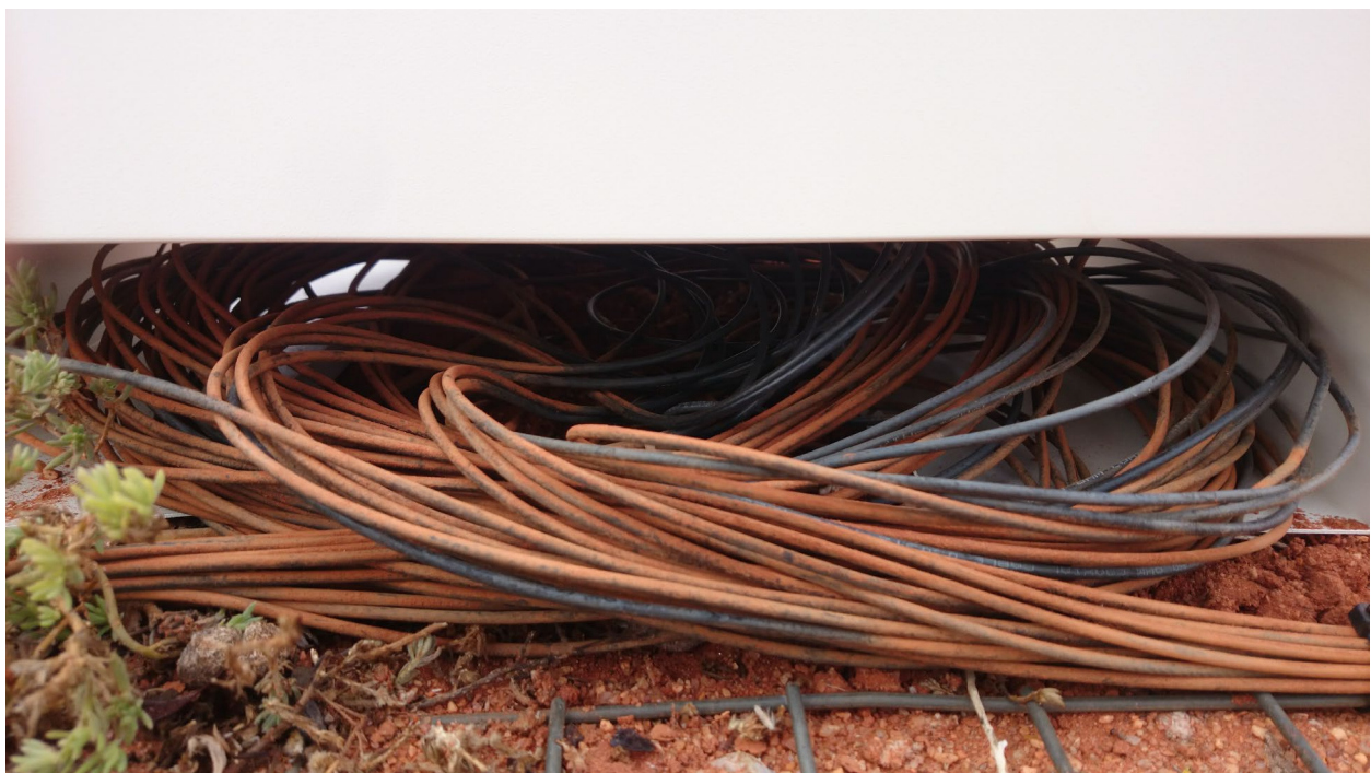
FIGURE 2: VIEW UNDERNEATH BEAM-FORMER SHOWING CABLE BUNDLING
